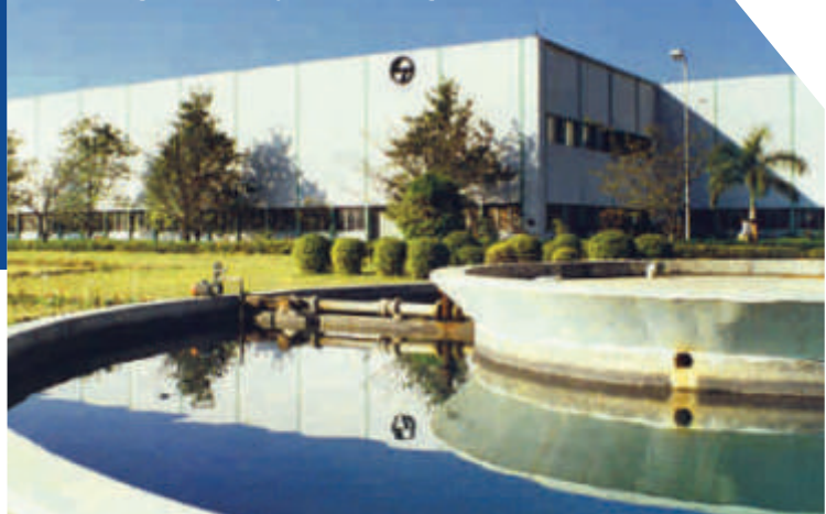
Switchgear Factory, Ahmednagar
