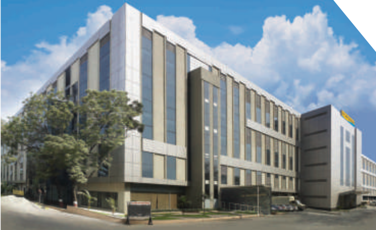
Switchgear Factory, Mumbai
